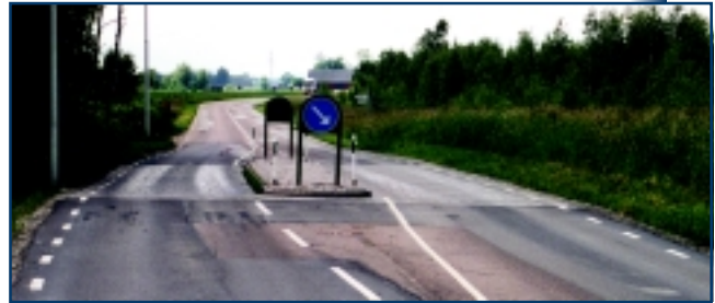
Figure 15. Example of gate with a platform, Sweden.
